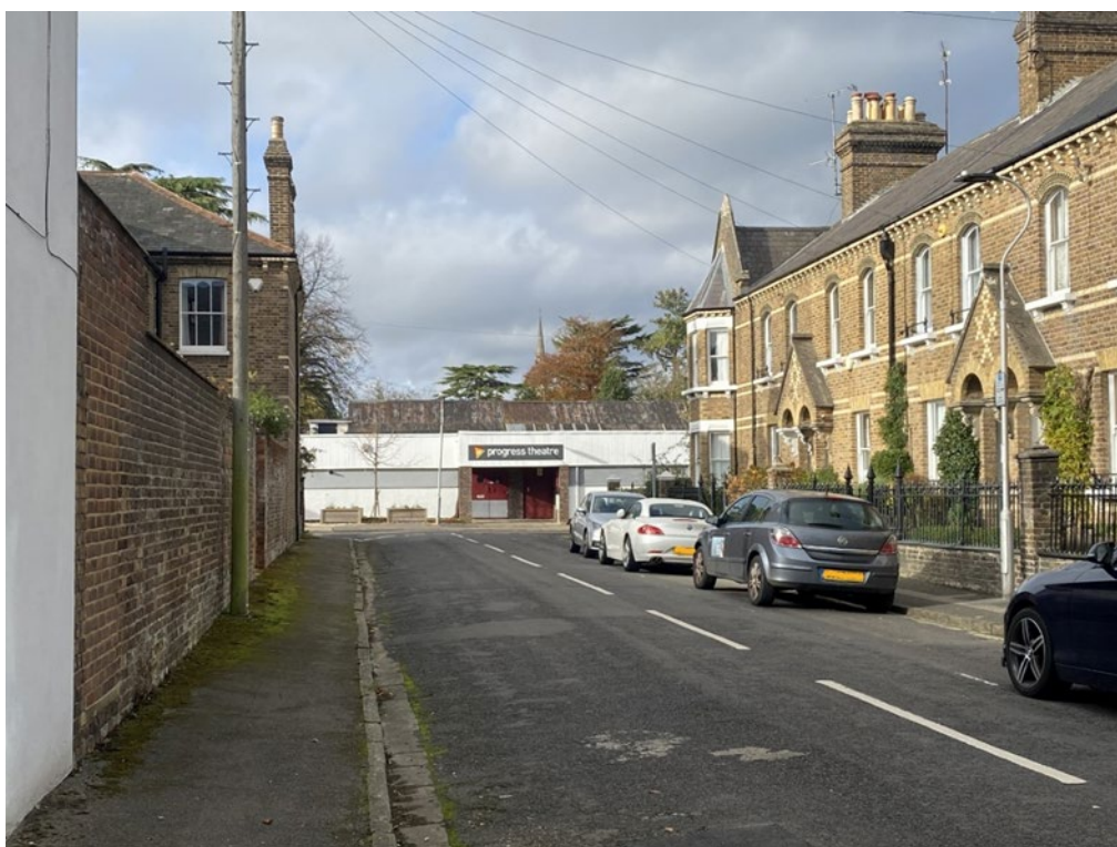
Figure 24: The Progress Theatre November 2025 (Image Claire Truman)
