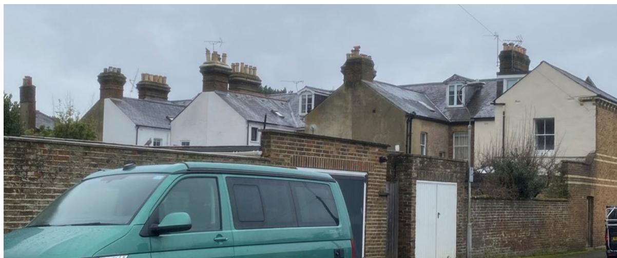
Figure 19: Original dormer windows to the rear of the north terrace of The Mount
