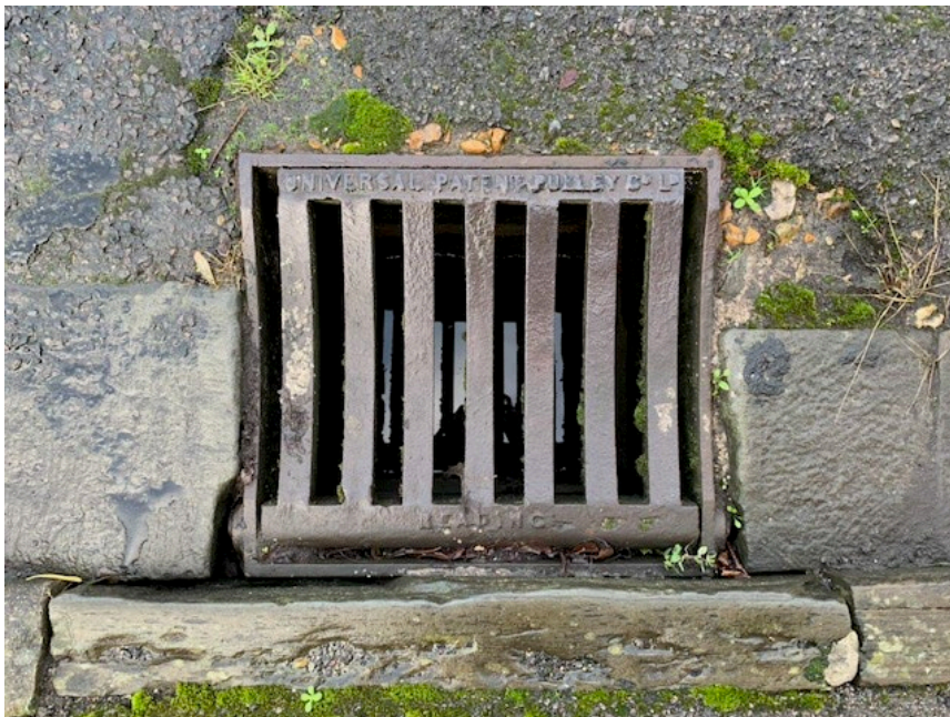
Figure 13: Universal Patent Pulley Co drain set within 'Caithness Flagstone Series' gutter and kerb stones (Image Evelyn Williams)
